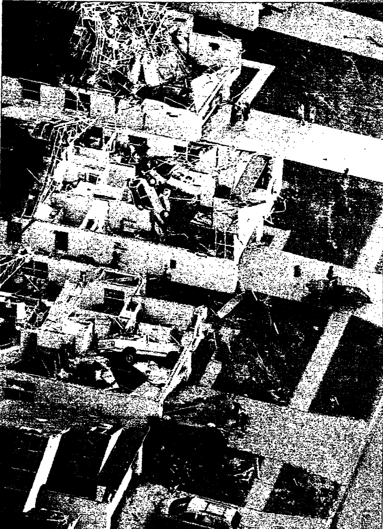
Residents return to survey the wreckage after a tornado had ripped through Kissimmee, south of the Disney complex
